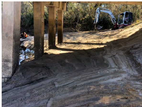
Bank erosion and scour repair: before and after
