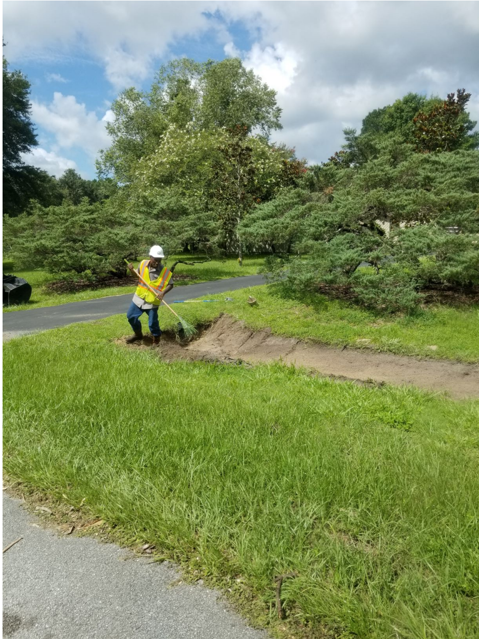
Ditch grading
