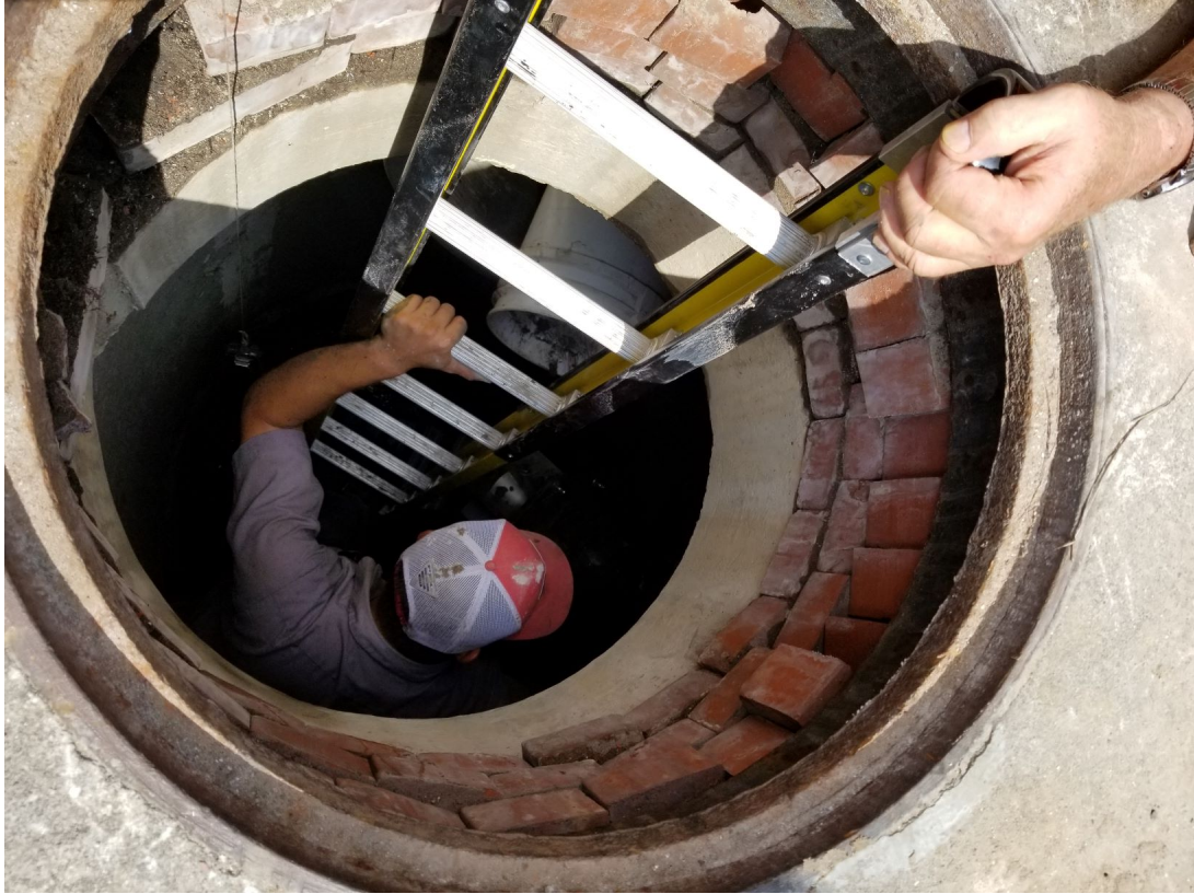
Connecting permanent piping from Robin
