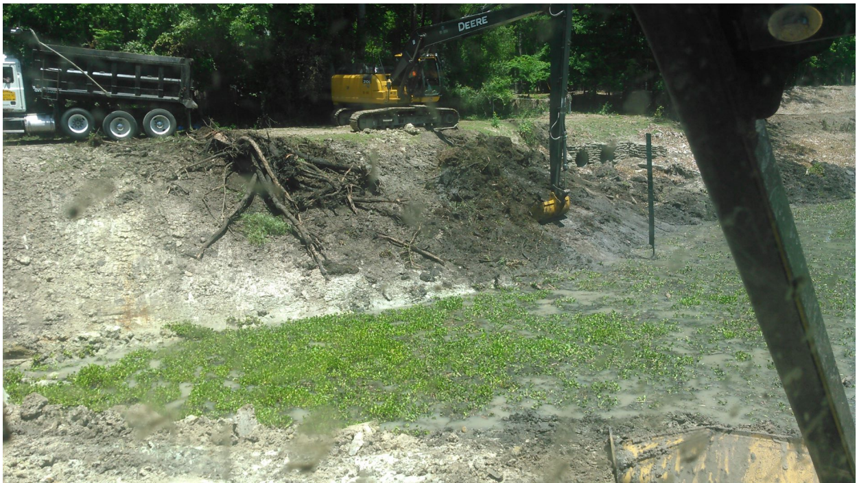
Dredging Robin Lane basin bottom
