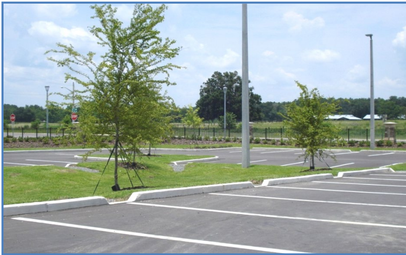
Curb cuts at Campus USA Headquarters in Alachua County allow runoff to flow into depressed island retention areas
