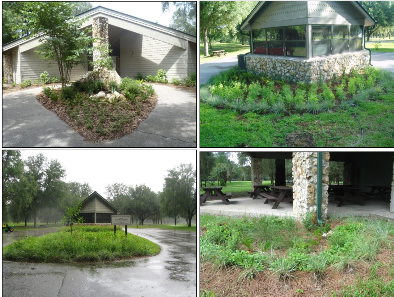
Figure 5. Clockwise from top left: planting at the lodge (July 3, 2013); wildflowers at the gatehouse (May 31, 2013); gatehouse landscape (July 21, 2013); and the rain garden (July 21, 2013).
