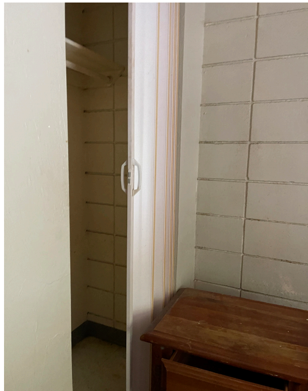
Figure 35 - CMU wall SW building
