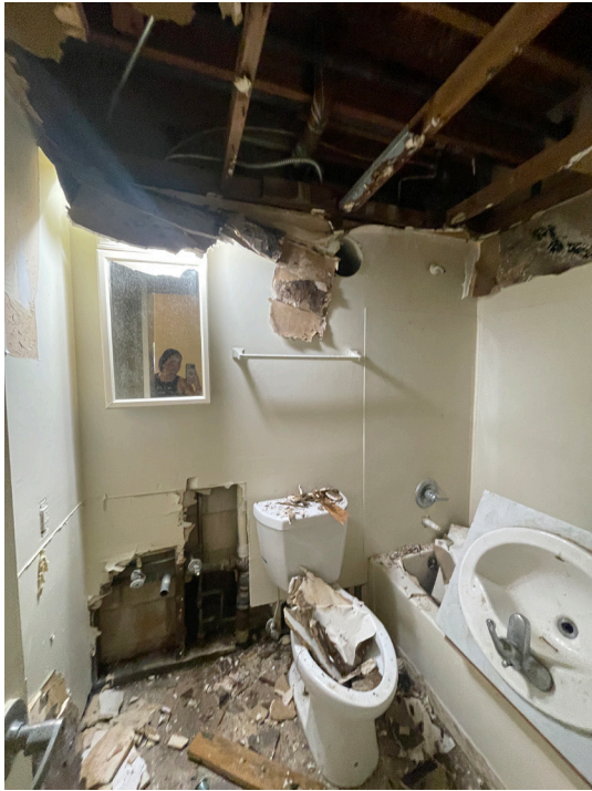
Figure 30 - Tore up bathroom in NE building
