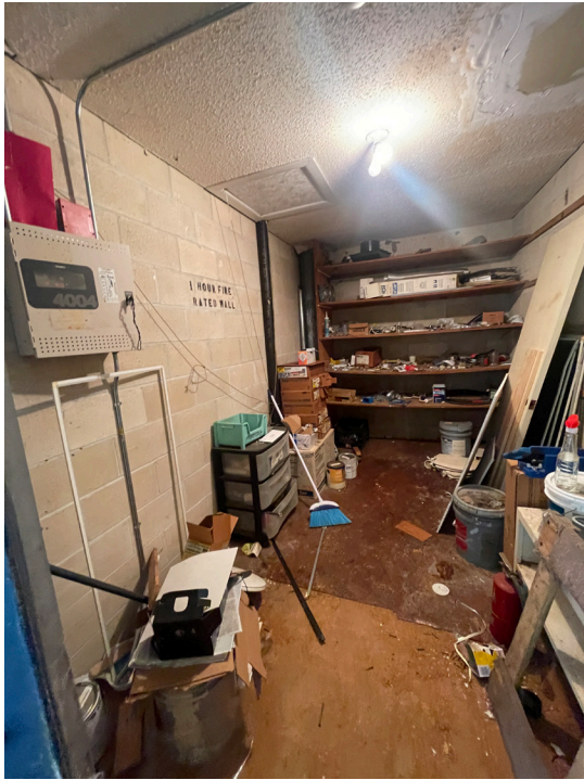
Figure 26 - Utility room interior
