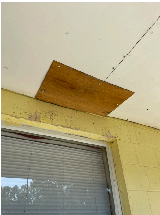
Figure 21 - Current condition of soffit in SW building
