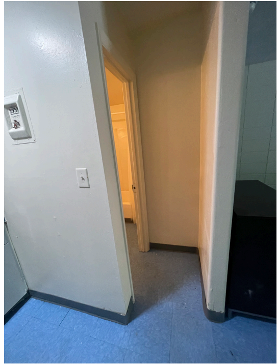
Figure 31 - Narrow bathroom door
