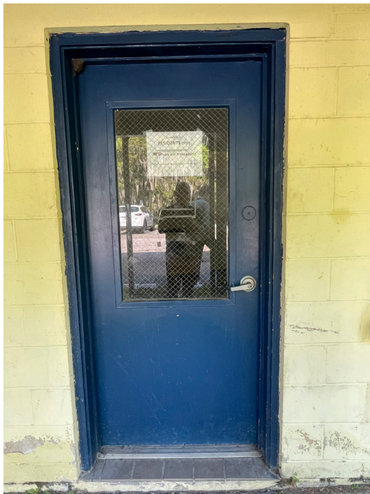
Figure 28 - Laundry room door
