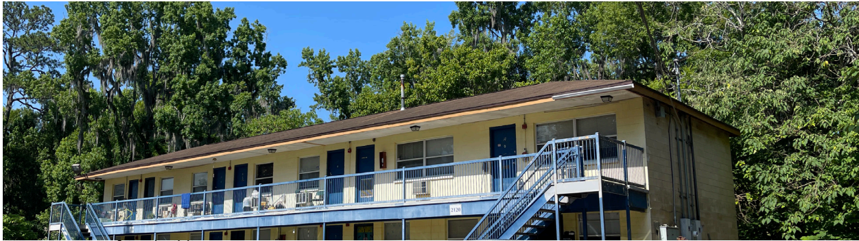
Figure 20 - Roof SW building
