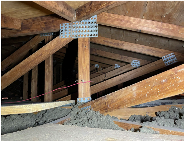
Figure 13 - Interior Roof NE Building
