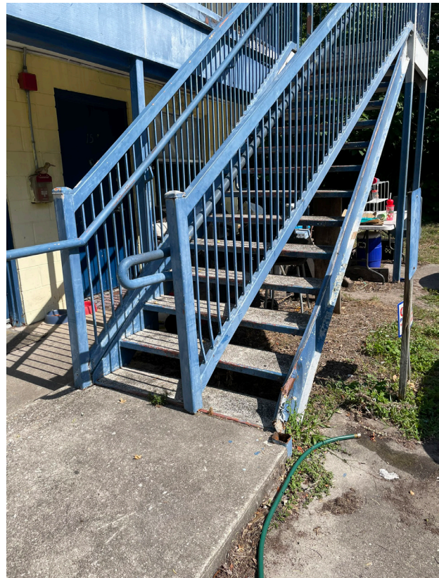
Figure 5 - Guard Rail SW Building
