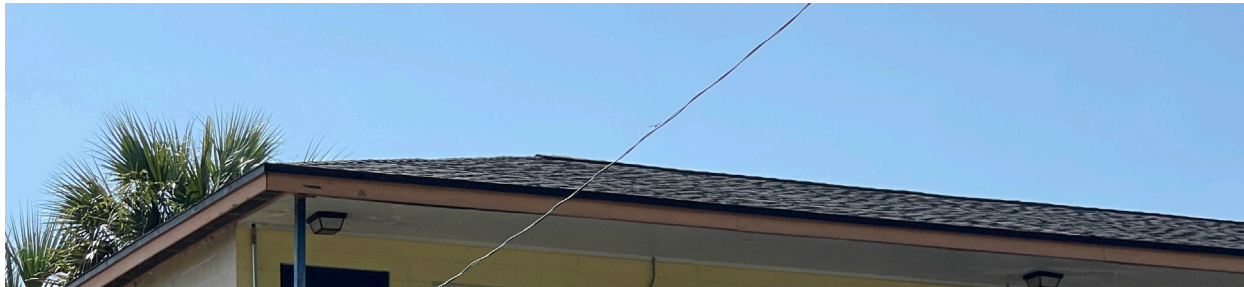
Figure 12 - Exterior Roof NE Building
