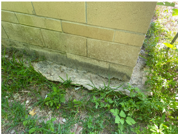
Figure 6 - Exposed Footing SW Building
