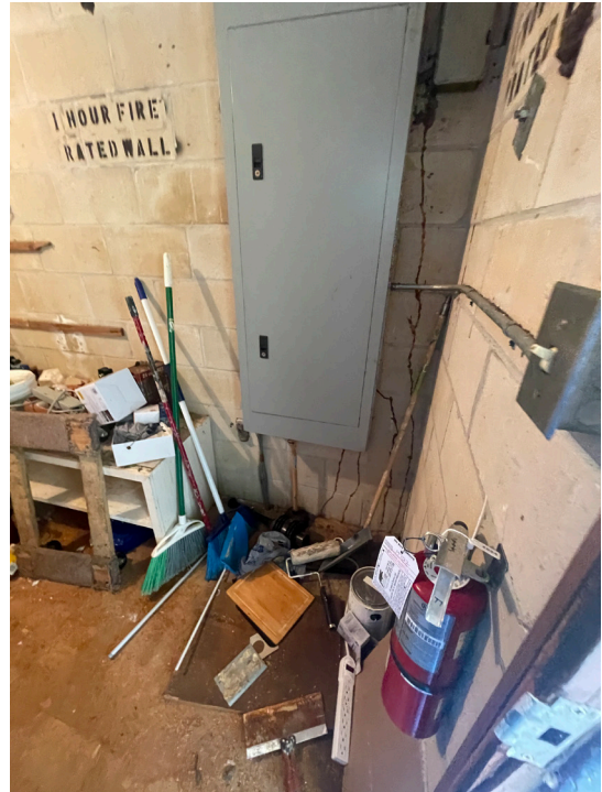
Figure 27 - Utility room interior
