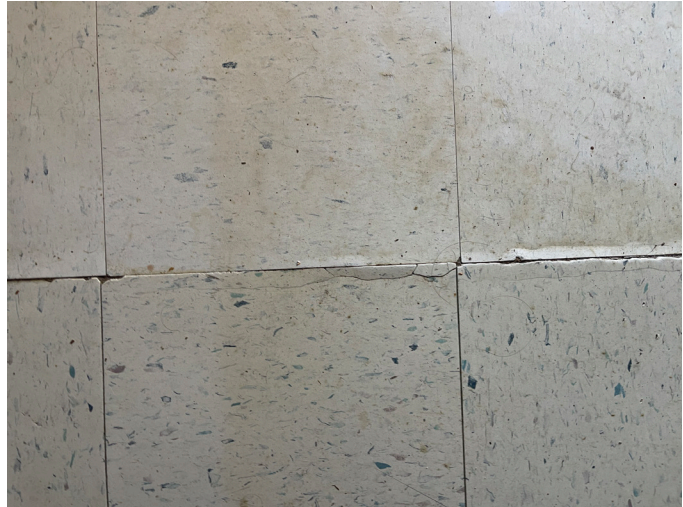
Figure 37 - Vinyl tile flooring
