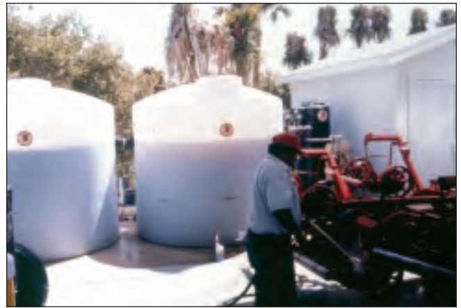
Figure 8: Recycling washdown system.
