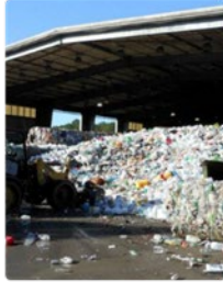
Materials Recovery Facility (Recyclables)
