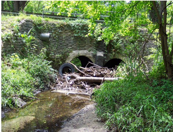
Sweetwater Branch at SE 4th Street.
