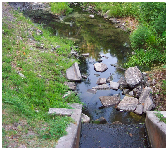
Sweetwater Branch at a culvert at SE 3rd
