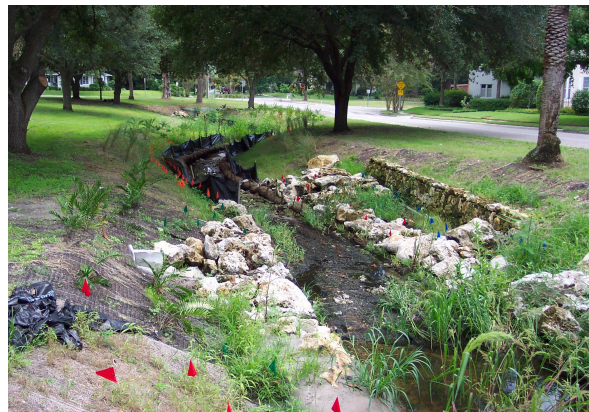
Restoration area on Sweetwater Branch upstream of the Duck Pond
