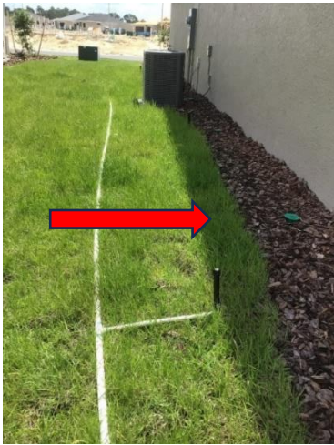
Above ground PVC pipe and emitters system used to establish turf (On Top of the World, Ocala, Florida).
