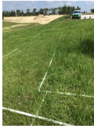
Above ground PVC pipe and emitters system used to establish turf (On Top of the World, Ocala, Florida).
