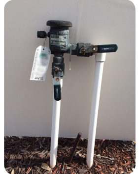
A backflow preventer and regular testing are required by law to prevent irrigation water from flowing back into our drinking water.
