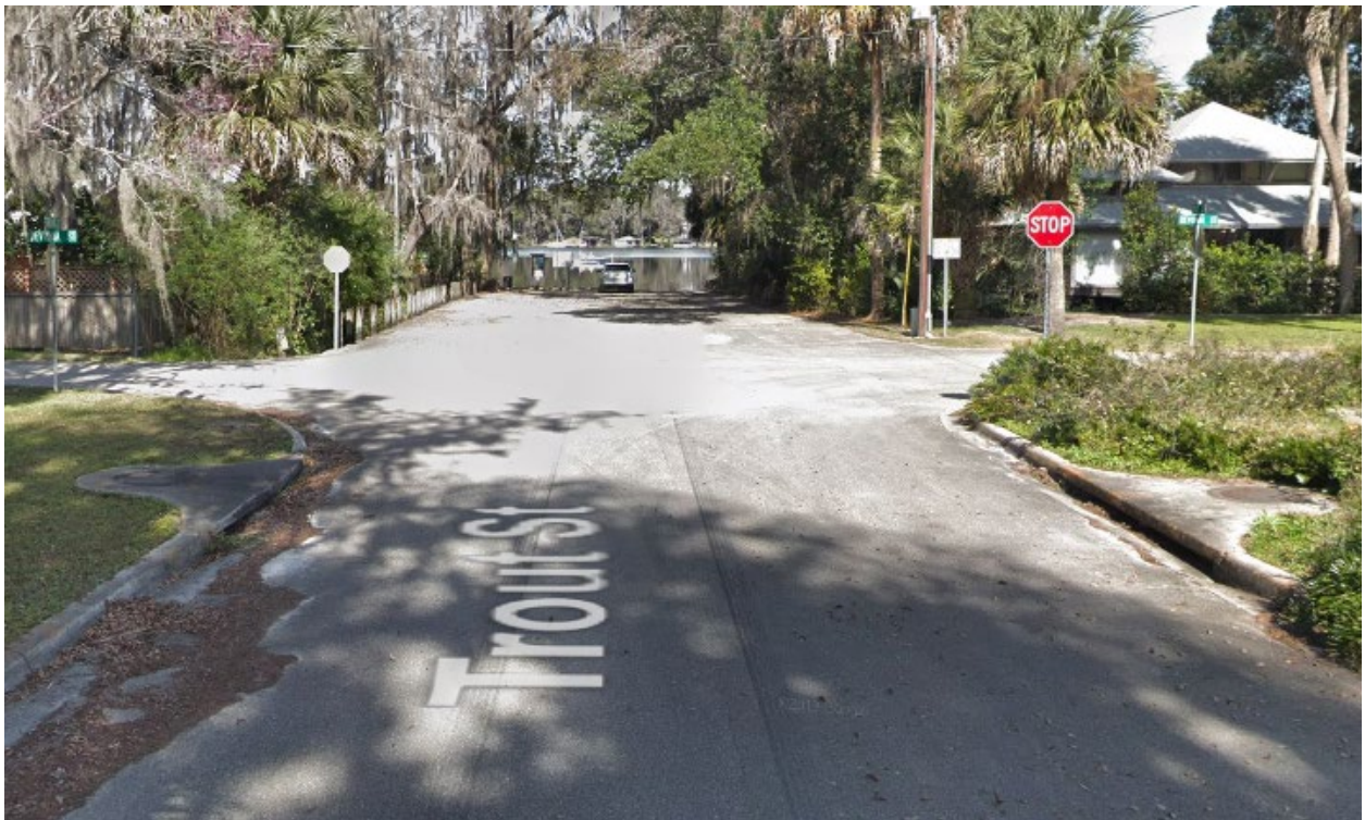
Figure 57. Stormwater drainage on Trout Street in Melrose, FL. Image is from Google Street View.
