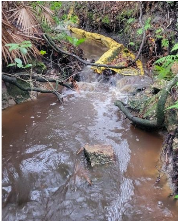
Figure 19. Flow in the southern culvert at NE 221 st Street.
