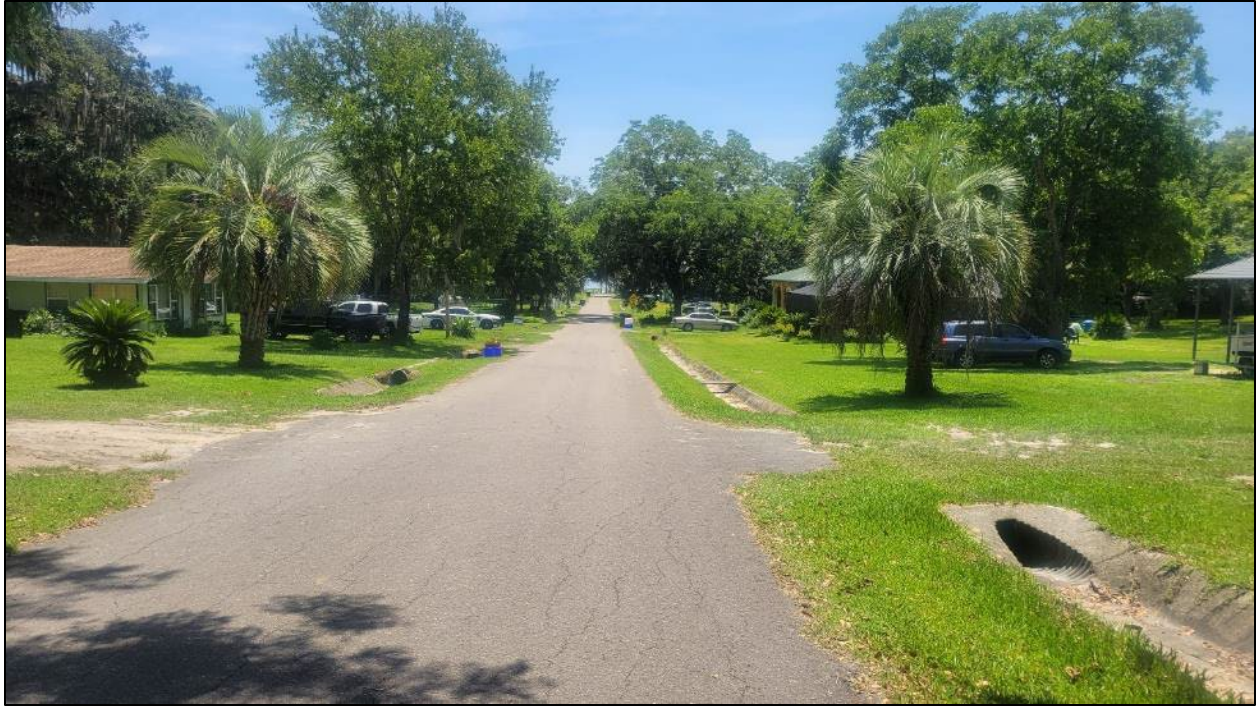
Figure 25. Stormwater collection system along NE 100 th Avenue.
