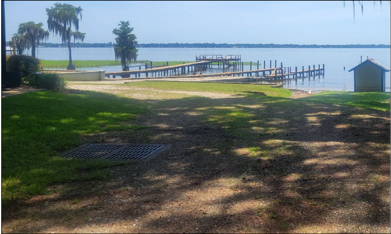
Figure 27. Outfall from the stormwater collection system along NE 101 st Avenue that discharges into Santa Fe Lake.
